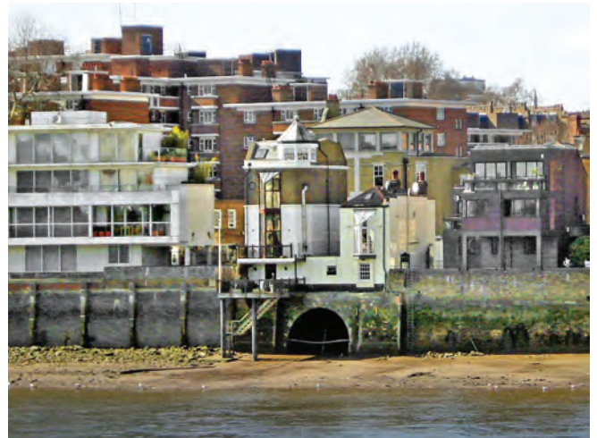
Tyburn Outfall, Pimlico. Photo by Diamond Geezer
